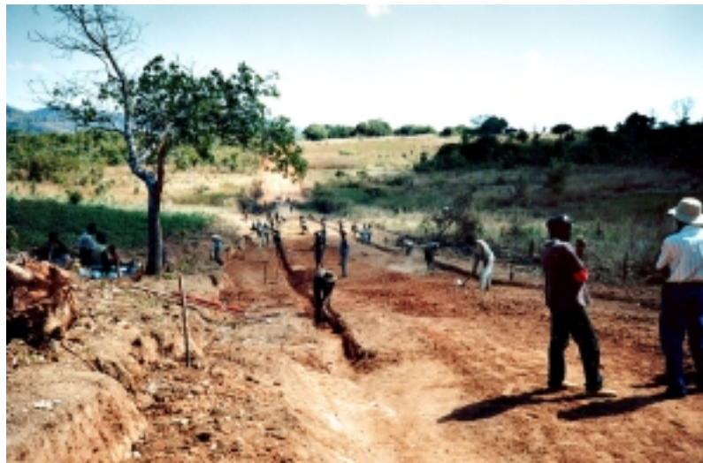
Figure 4: Labour Based Road Rehabilitation
