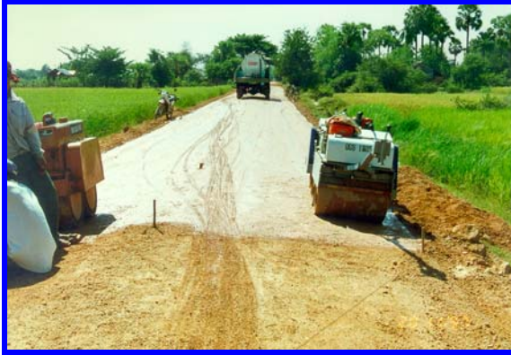
Image 10: Placement of Sand Sub-base Compaction of Sub-grade and Sub-base Layers
