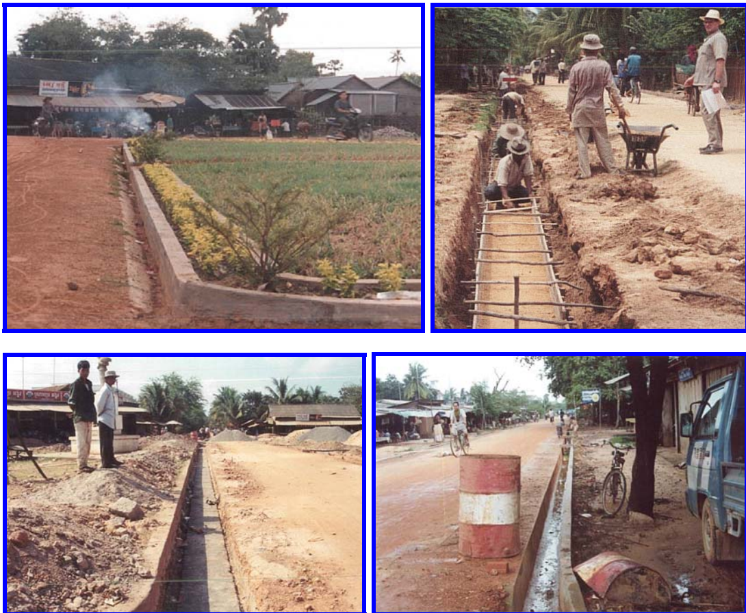
Images 20 - 23: Drainage Works
