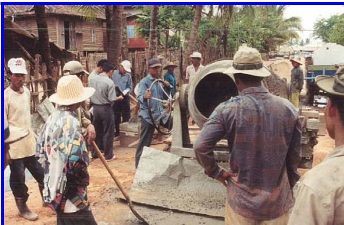
Image 13: Mixing of Concrete
