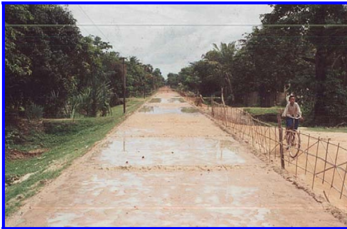
Image 19: Curing and Protection of Concrete
