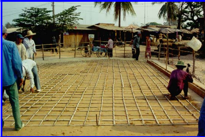
Image 12: Placement of Bamboo Mesh, wooden spacers to be inserted under mesh
