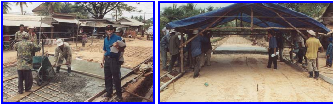
Images 14 & 15: Placement of Concrete and Sun Shelter
