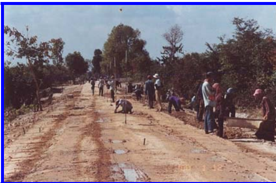
Image 9: Setting out of road alignment and level
