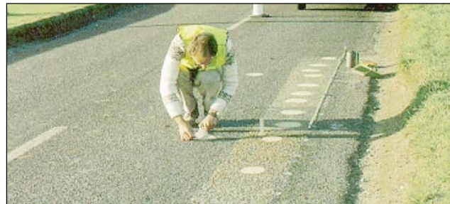
Measuring texture depth of trial panels by sand patch method
