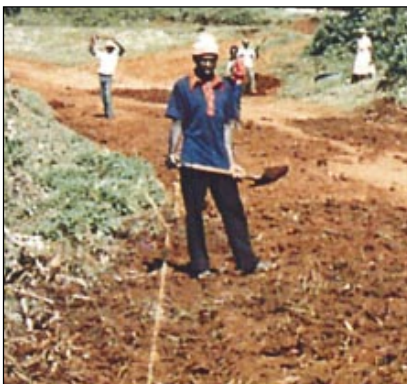
Re-shaping of road profile using simple handtools
