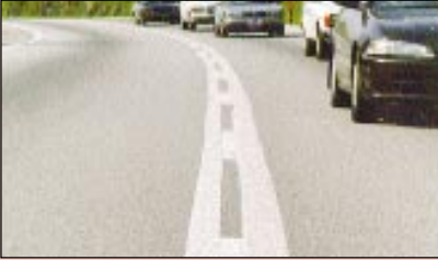
Centre-line road marking trial
