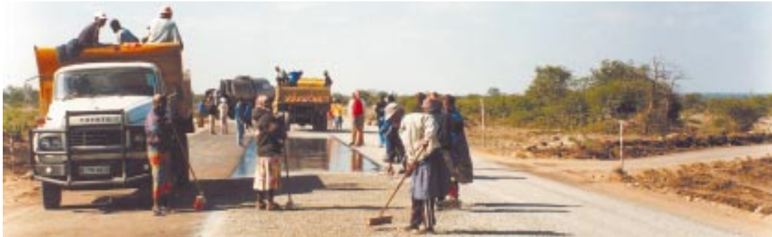
Surfacing a low volume road in Southern Africa using an Otta seal
