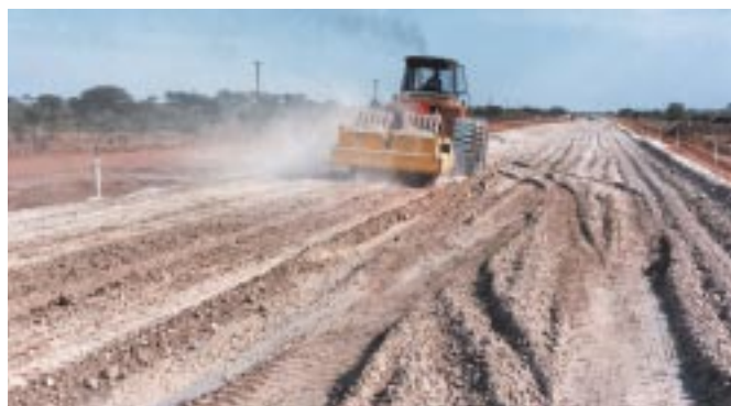
Constructing roads with calcrete, Botswana
