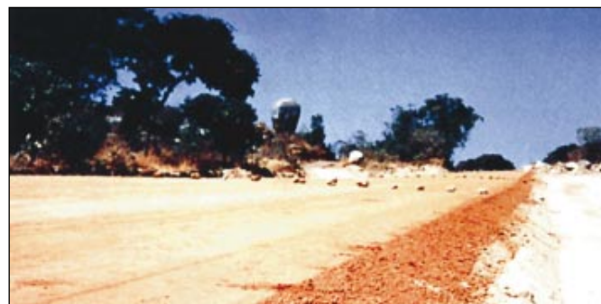
Low grade lateritic gravel roadbase in Zimbabwe
