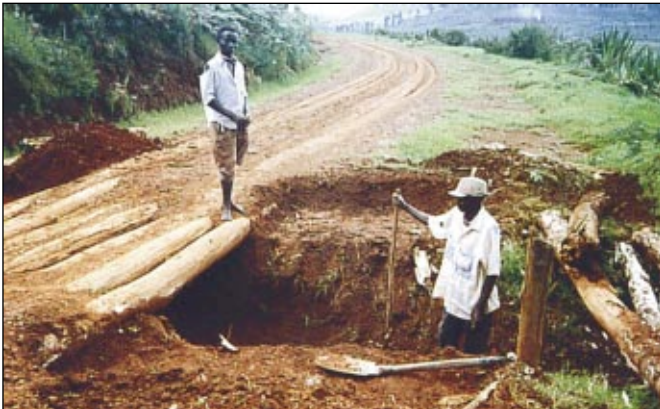
Reconstruction of culvert, Democratic Republic of Congo
